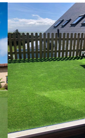
51 - 52 Roof Artificial Turf
